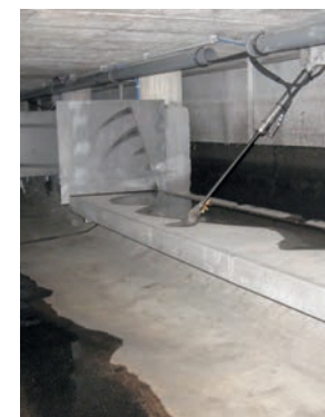
ESK-Weir with hydraulic drive
